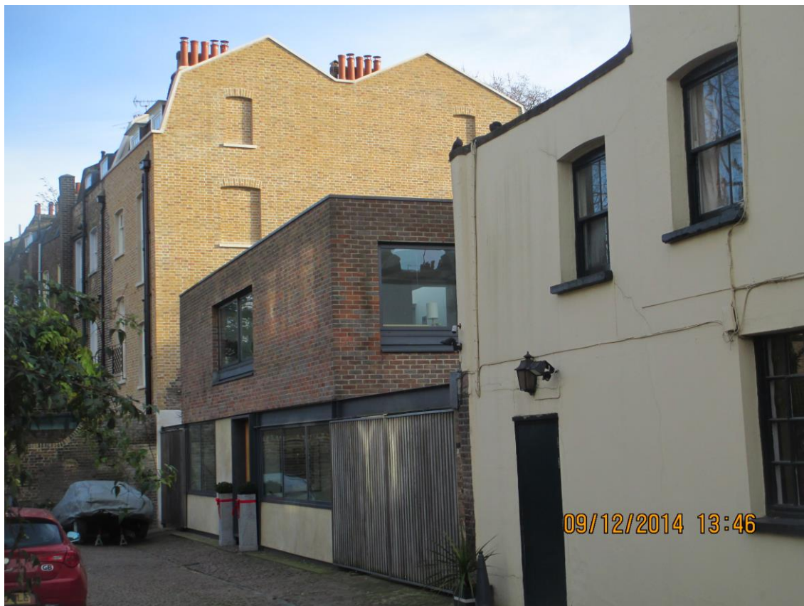
Image 4 – View of front elevation from Compton Avenue
