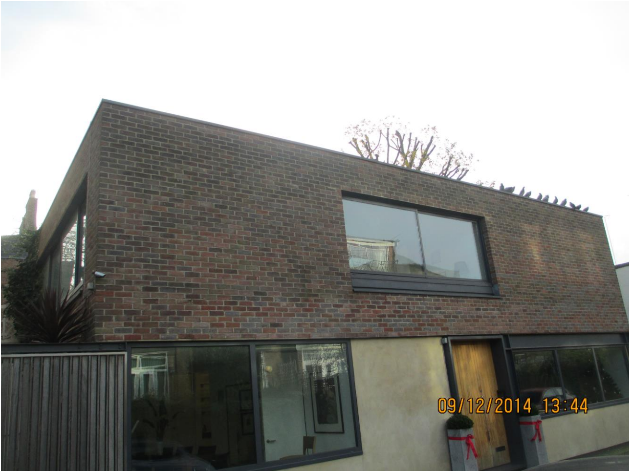
Image 3 - View of front elevation of site
