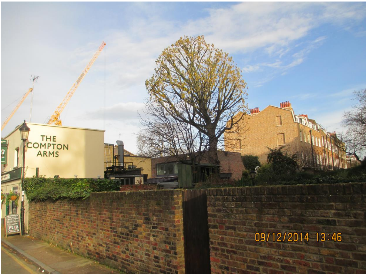
Image 6 – View towards the rear elevation from Compton Avenue
